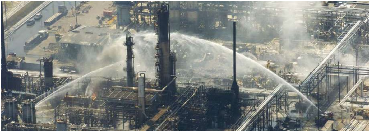
Fire following explosion at Texas Oil Refinery, 2005. Courtesy Chemical Safety and Hazards Investigation Board
