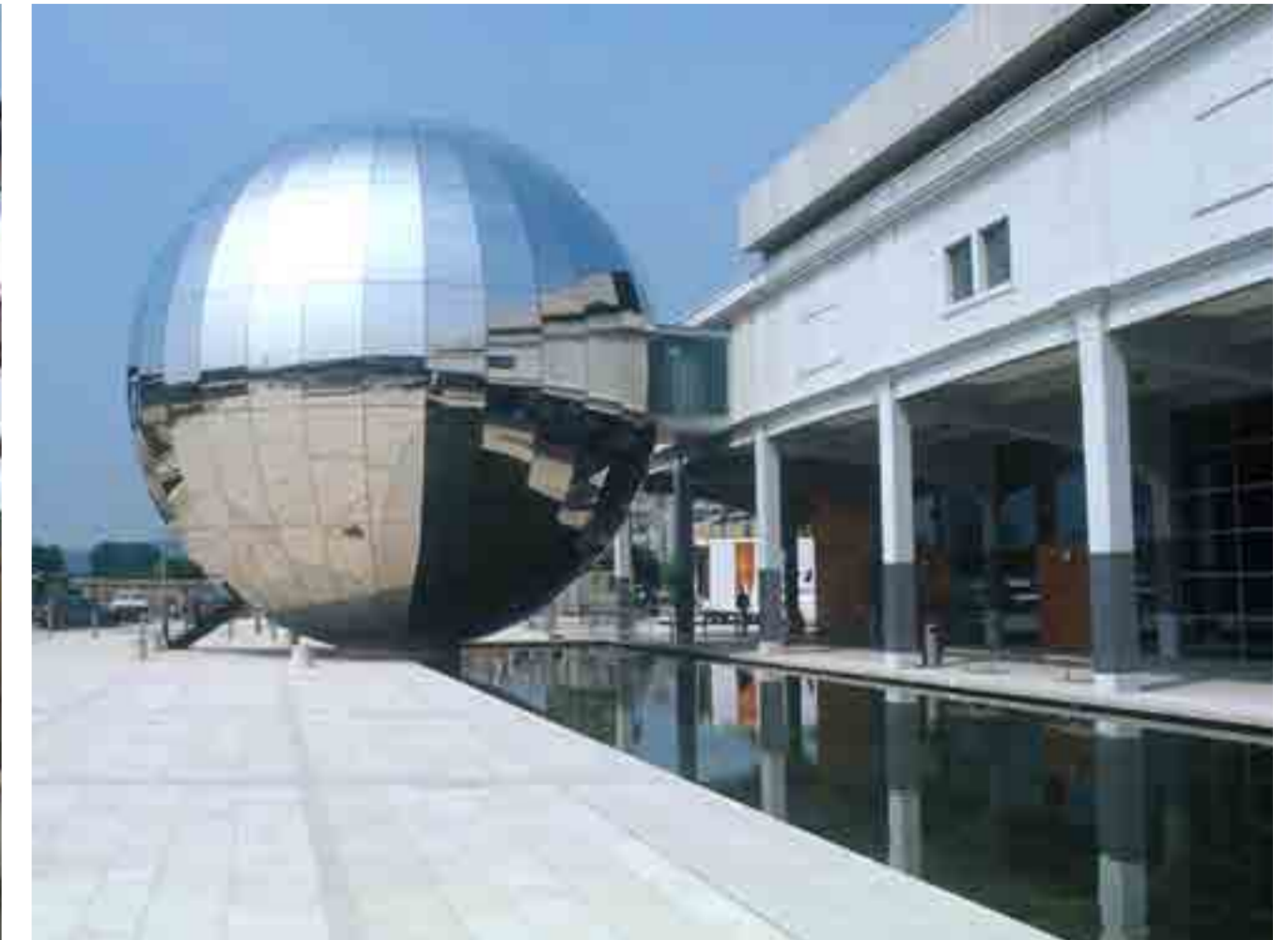
Explore@Bristol Refurbishment, alteration and extension of a Grade II listed building
