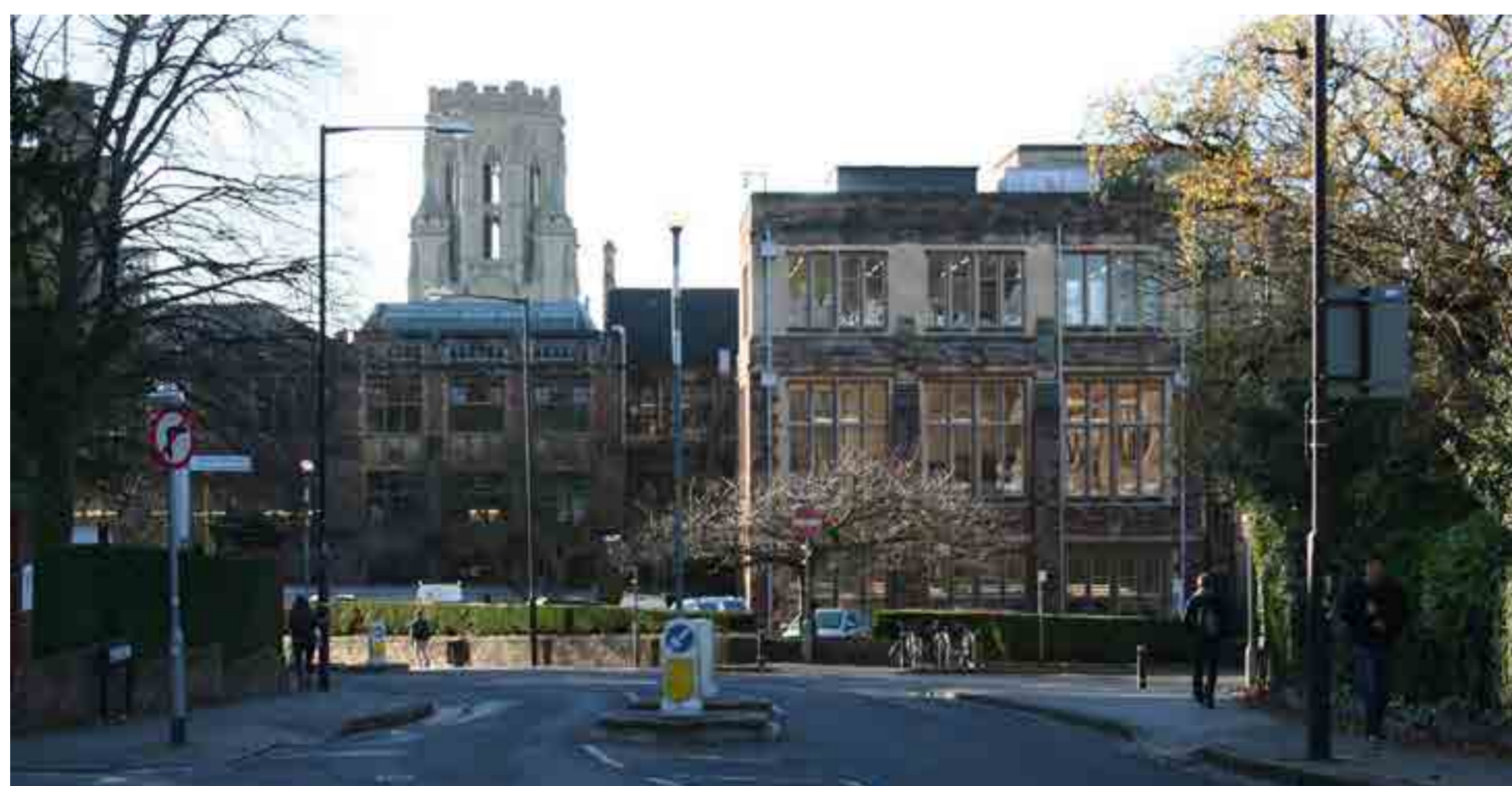
View of the Fry Building from the north with the Wills Memorial Tower beyond
