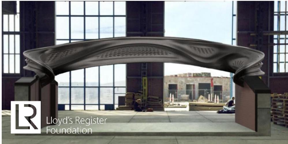
**Digital twin** of world's largest 3D printed structure to inform design, track performance, and feed into future 3D structures
