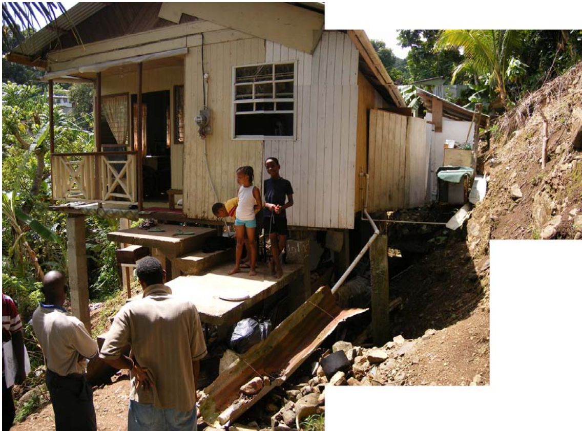
Fig. 4 Typical wooden house reconstructed (on its original site) after damage by a landslide in the cut slope above
