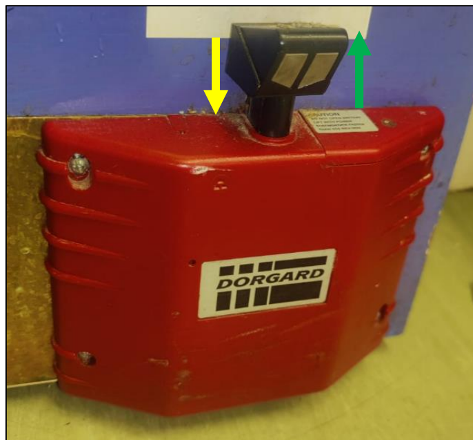
Photo of Dor Guard. Yellow arrow indicates direction to push black button to prop open door, green arrow indicates direction to release Dor Guard, thus allowing the door to close.
