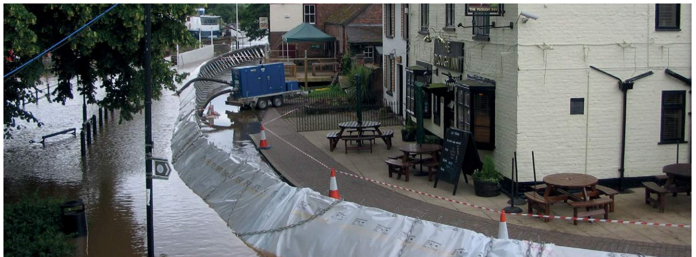
Temporary flood defence structures at Upton-on-Severn in the summer of 2007.
