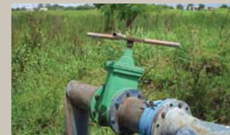
Top: Robert Cottrell and Hayley Sharp, members of the EWB-UK Bristol team that took part in the Havana project, which saw students from EWB-UK working to improve Havana's water supply, bottom: an inlet valve in Havana
