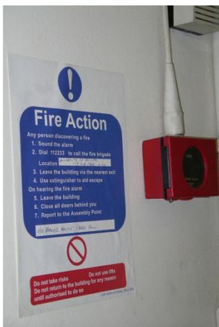
A Fire Action Notice located correctly adjacent a red manual call point. Two area of the sign need to be completed by providing information on:
