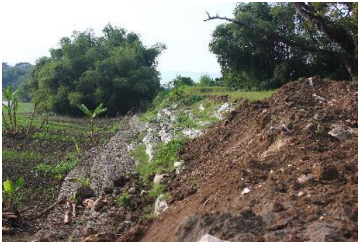
Gabion and sand-bags for slope protection
