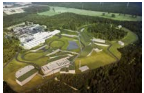
Figure 6: GSI accelerator facility
