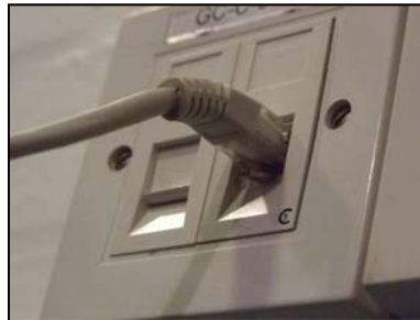
A ResNet socket with network cable connected
