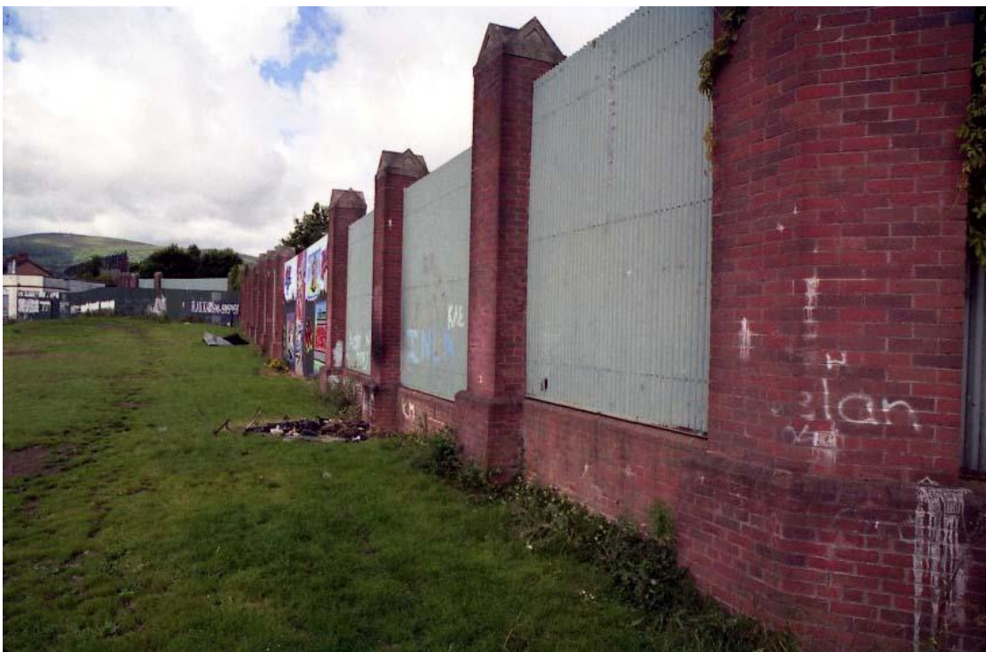
Fig. 1.2 A five metre high brick wall with reinforced steel panels runs along the back of properties from Ardoyne Road to Deerpark Road. Interface Map No.4 . Image courtesy of Frankie Quinn, © Belfast Interface Project.
