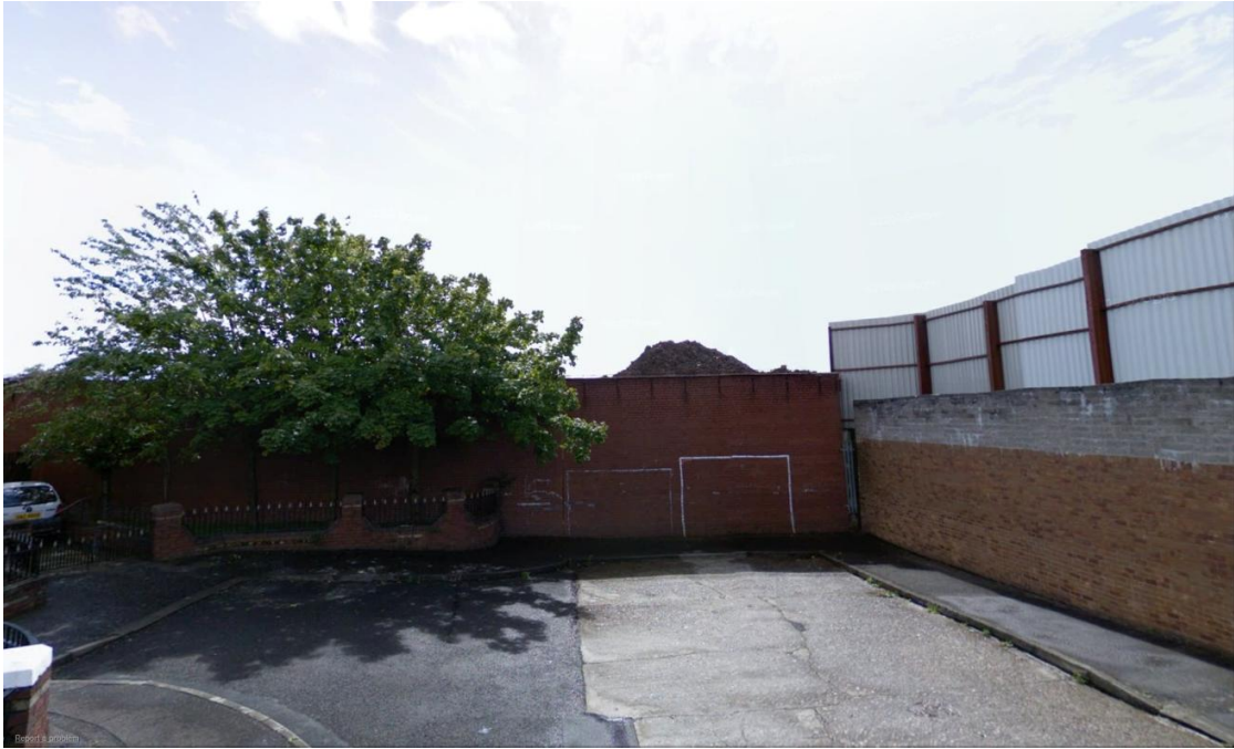
Fig 1.5. A brick wall, reinforced with steel fencing, obscures the line of sight from Antigua Street to Crumlin Road. Interface Map No. 6
