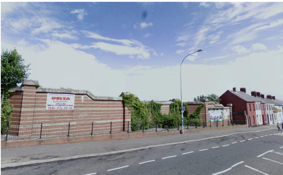
Fig 1.4 A newer looking brick wall, built in the 1990s, runs along Oldpark Road. Interface Map No. 7
