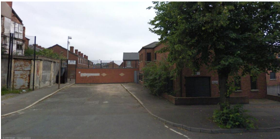
Fig. 1.11 A brick wall restricts access between Duncairn Gardens and Hallidays Road. A metal gate provides pedestrian access. Interface Map No. 14
