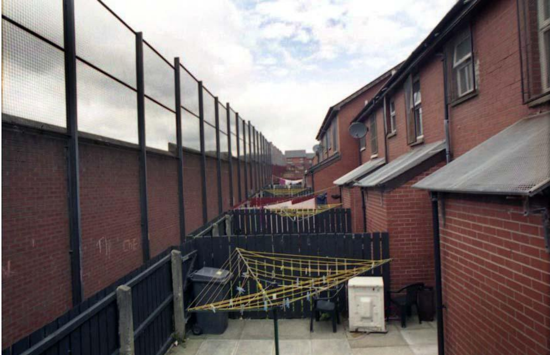
Fig 1.3 A brick wall reinforced with steel mesh runs along the back of houses on Rosevale Street. It continues out of shot along Rosapenna Street and Oldpark Road. Interface Map No. 10. Image courtesy of Frankie Quinn, © Belfast Interface Project.
