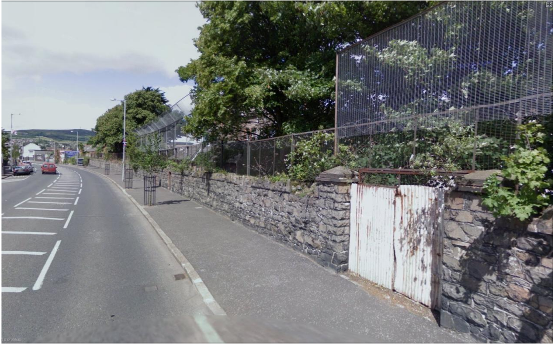
Fig. 1.6 A low brick wall and gate reinforced with steel mesh obstructs the line of sight between Brompton Park and Twaddell Avenue. Interface Map No. 3
